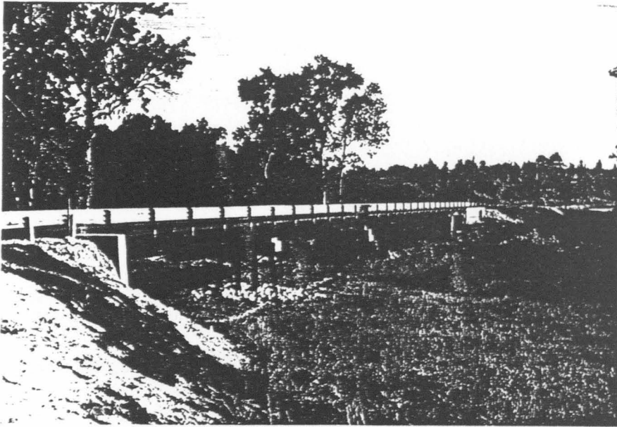
a) overall view of Wittson Bridge
